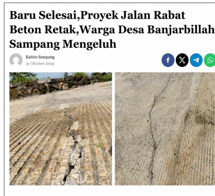
Figure 4. Road Infrastructure After Construction
