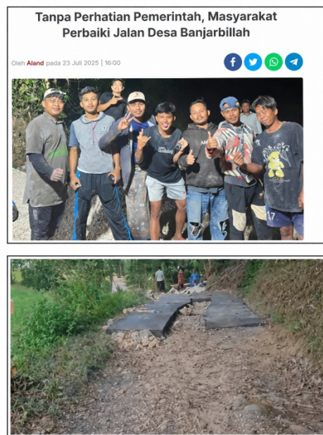
Figure 3. Community Initiative to Repair Damaged Roads in Banjarbillah Village
